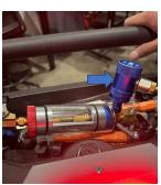
OPEN the valve on the incoming flow side (RED cap side on Mastercool sight glass) to allow freon to flow through the unit. The valve lever will be straight indicating that the valve is open
